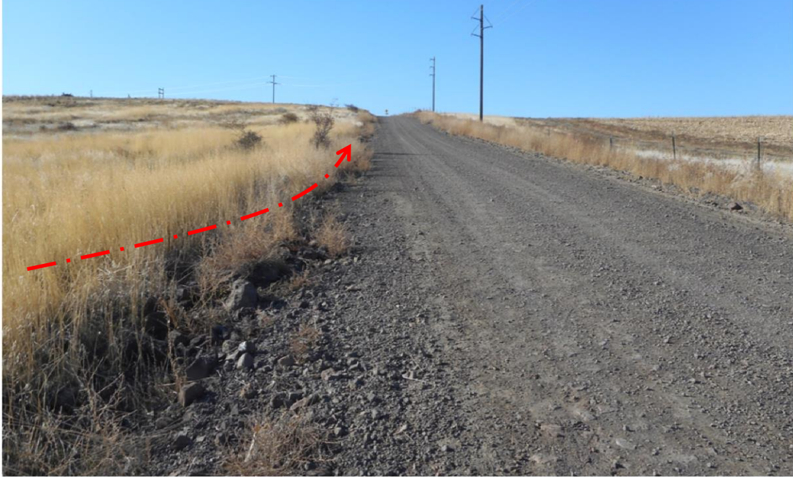
AT STATION 24+00 LOOKING SOUTHWESTERLY ALONG CENTERLINE
