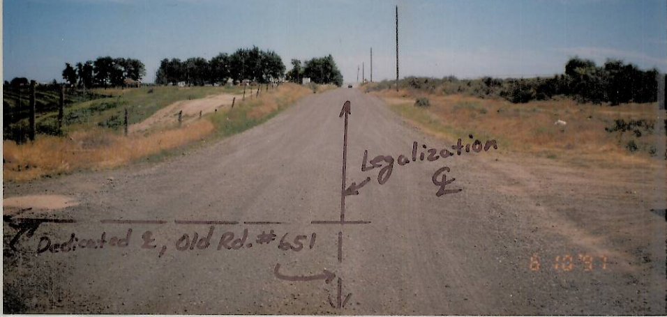
Station 106 near west end of Legalization looking East.
