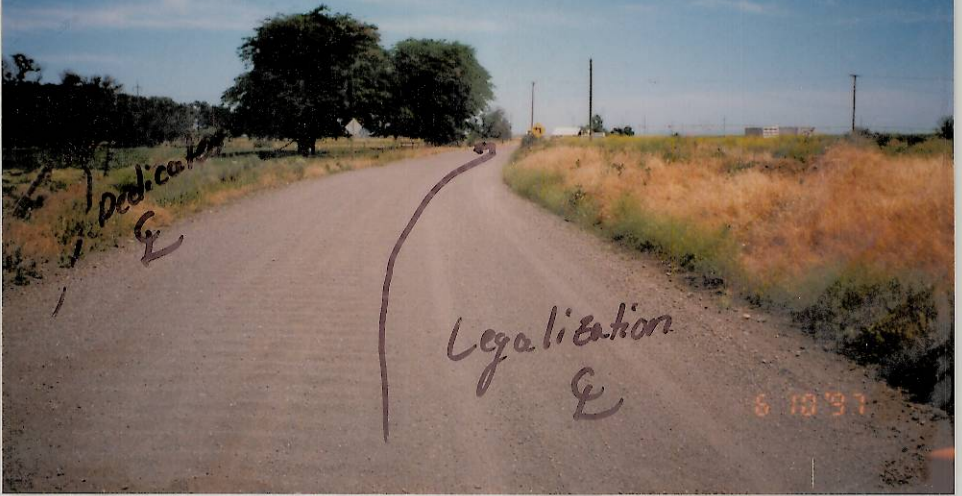
Station 156 Looking Northeast
