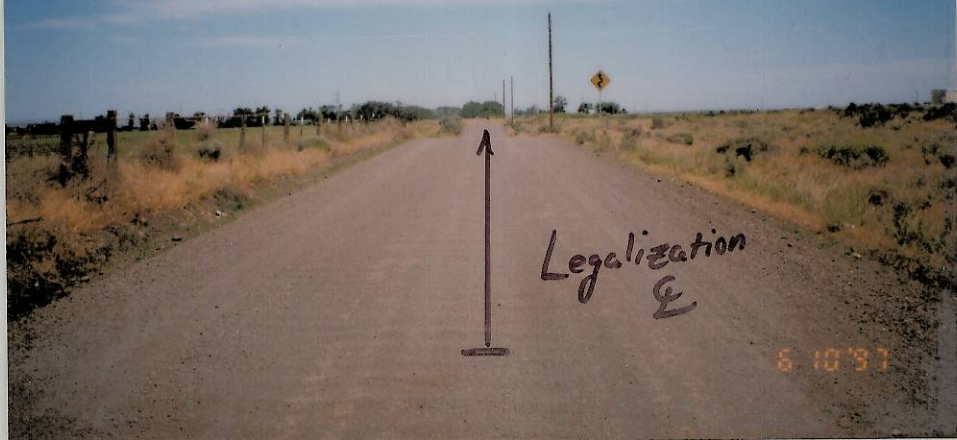
STATION 133 Looking Northeast.
