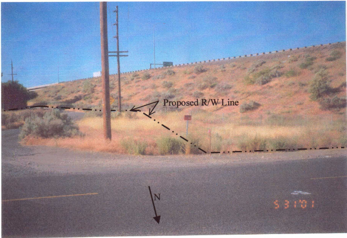
AT 3 RD STREET LOOKING SOUTH
