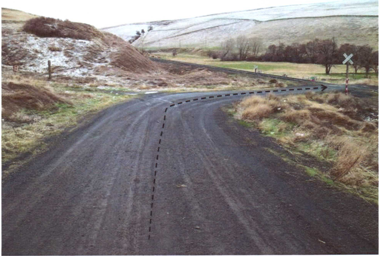
STATION 3+50 LOOKING SOUTHWEST
