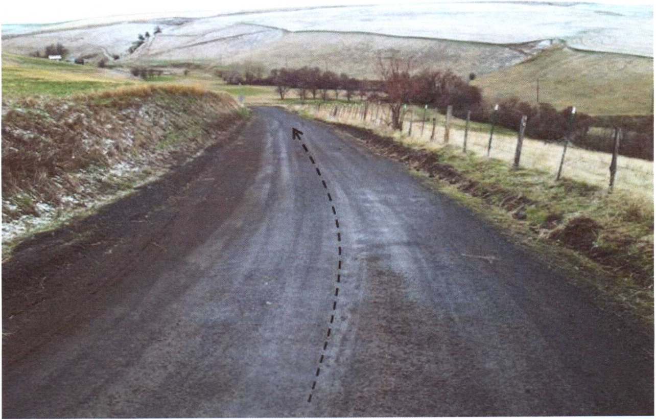
STATION 13+00 LOOKING SOUTHWEST
