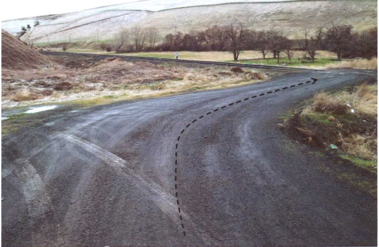
STATION 2+50 LOOKING SOUTHWEST
